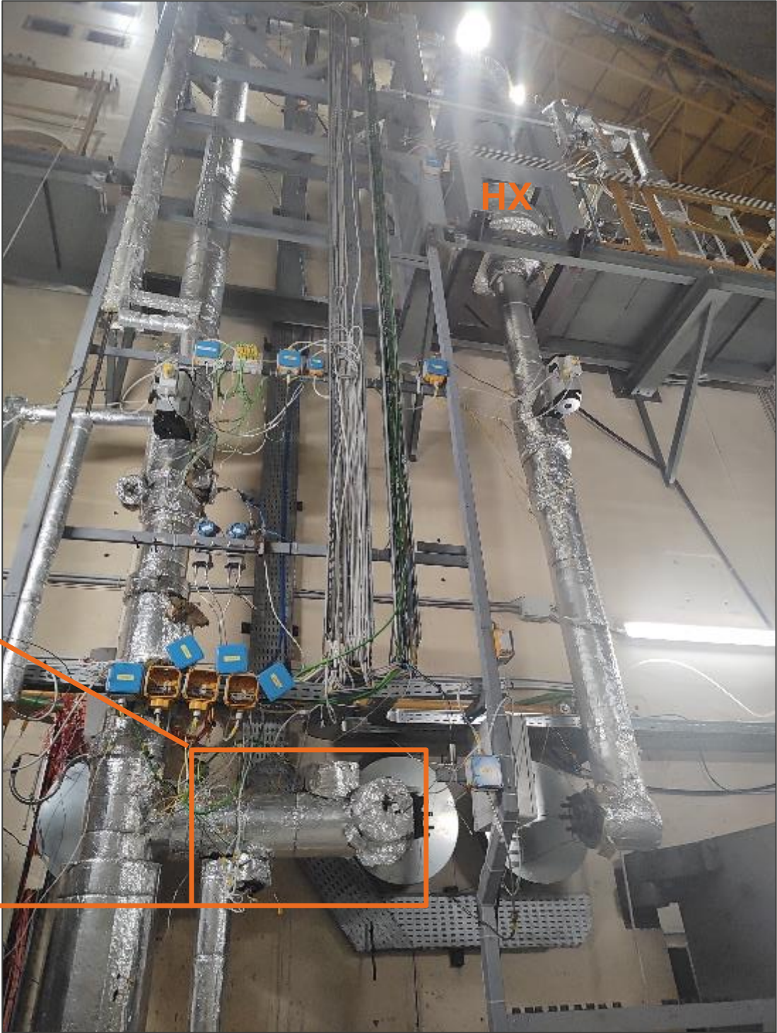
TEST SECTION (replacing existing piping)
